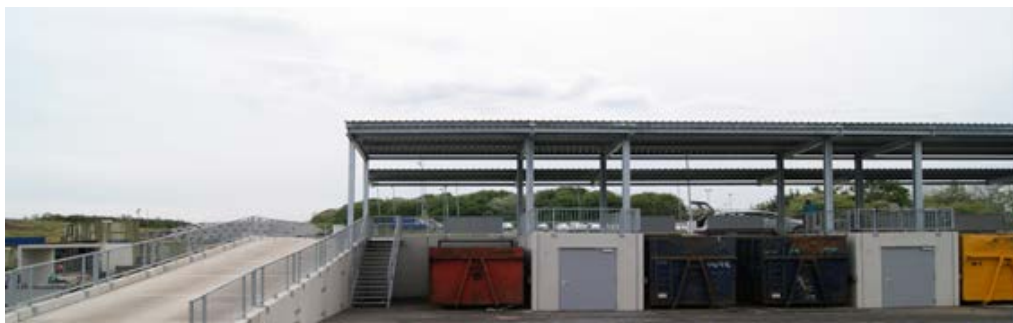
15. Example of a Modulo Beton raised level HWRC at Lamby Way
